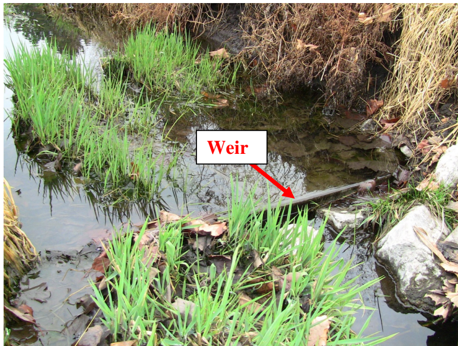
Figure 3.4: Photograph of the weir at Taylor Park (looking upstream)
